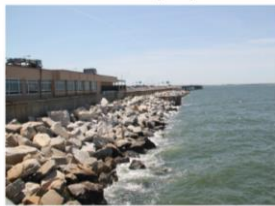
Sea Wall and Riprap
